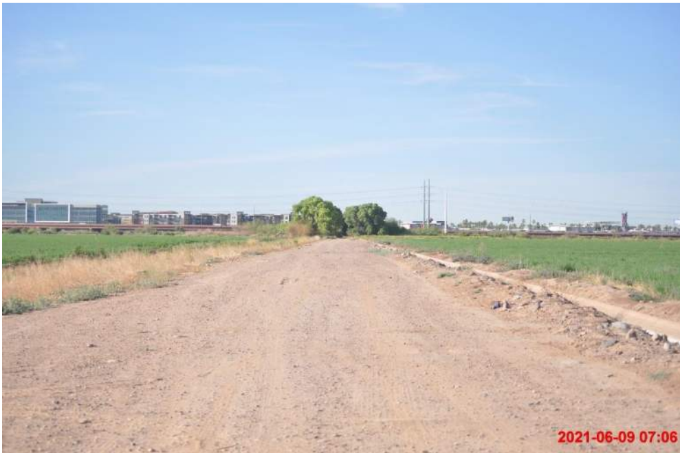
View of 84 th Street alignment looking south.
