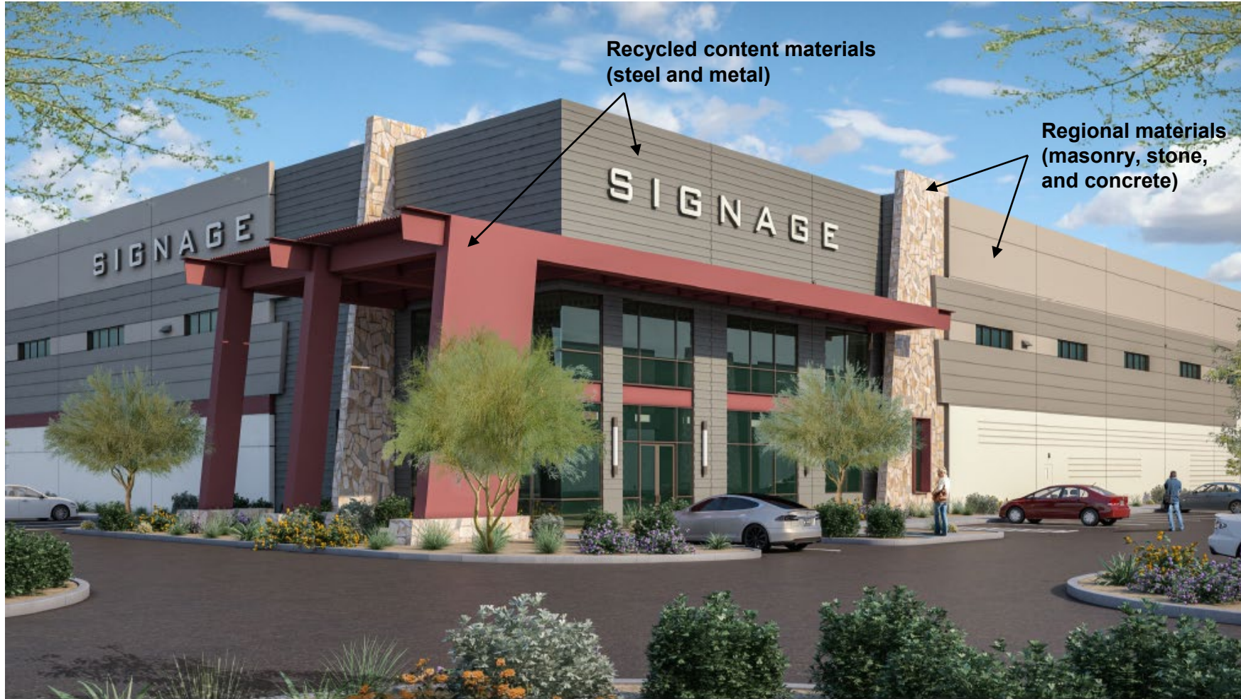
Core and Shell building
