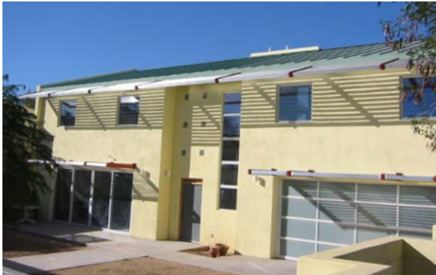
McDonnell Infill Office/Residence
