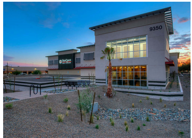
Utilize LED lighting with a warm color temperature
