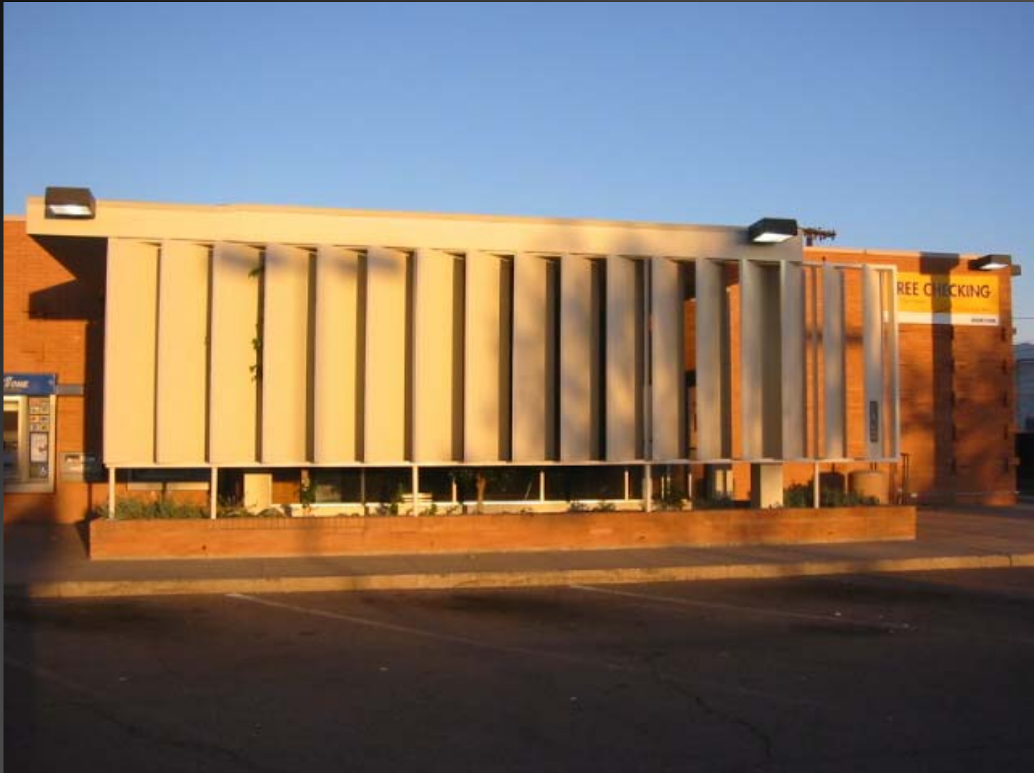
West Elevation at Bank One Phoenix
