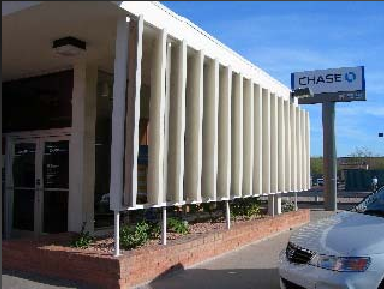
West Elevation at Bank One Phoenix
