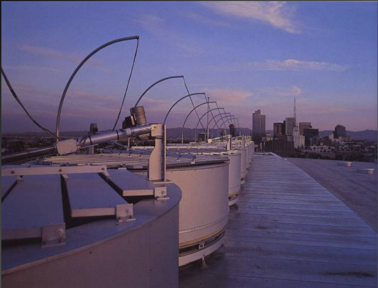
Louvered Skylights, Phoenix Central Library Will Bruder Architects
