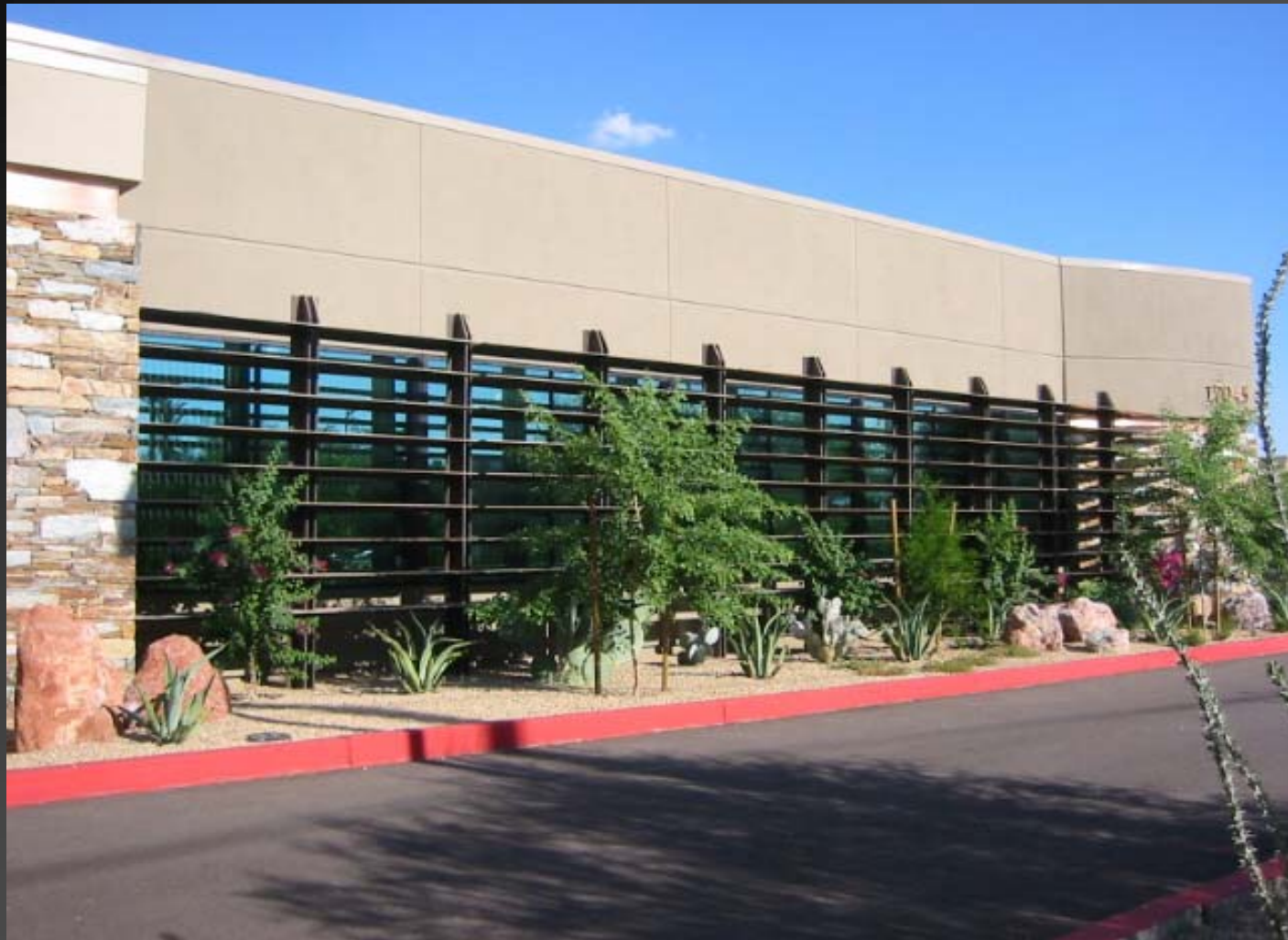
Louvers (mini-overhangs) on West Elevation in August
