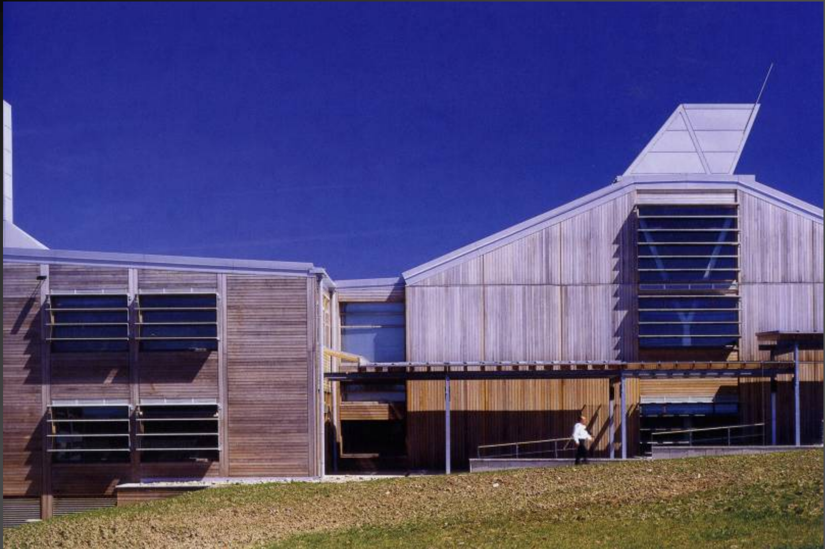
East and west facade - Arup Campus, Solihull, UK (Arup Associates, 2001)
