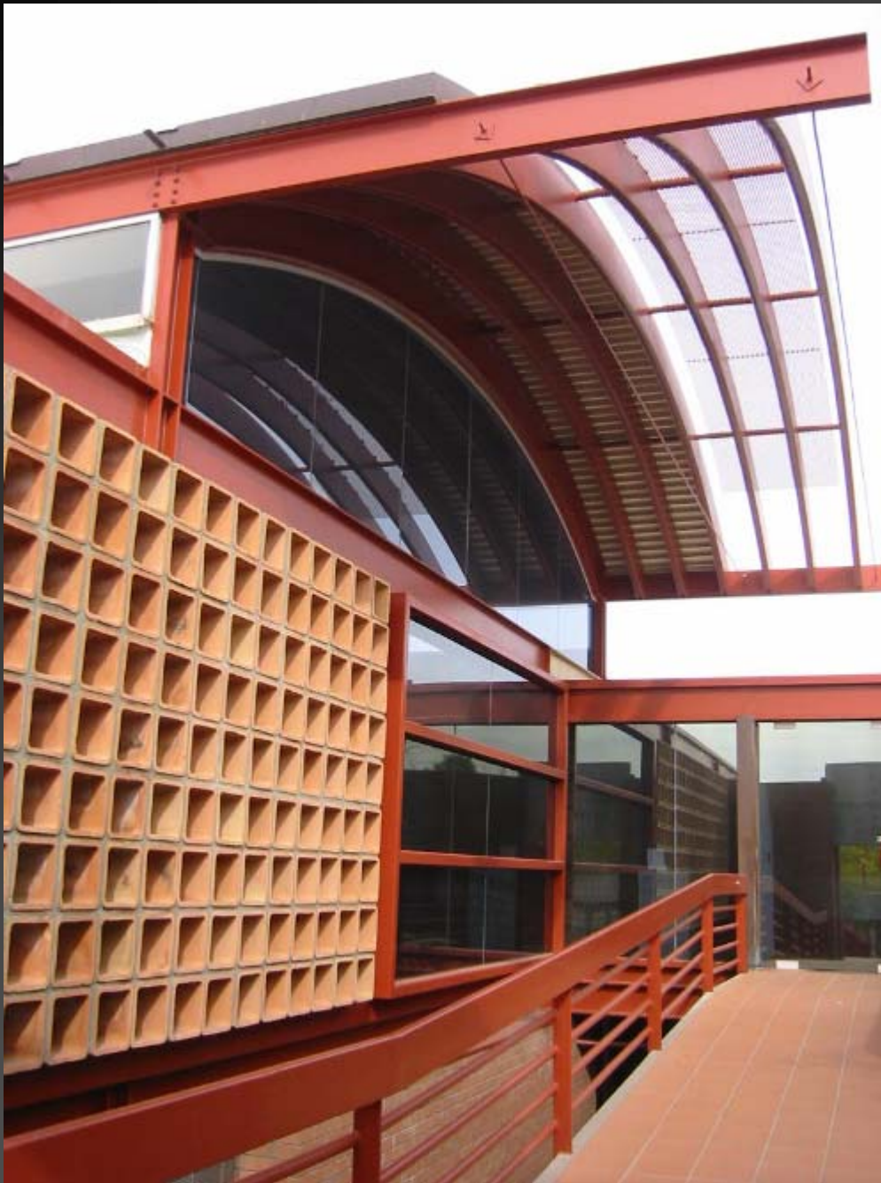
South facade AZ Cardinals Training Facility (Jones Studio, 1988)
