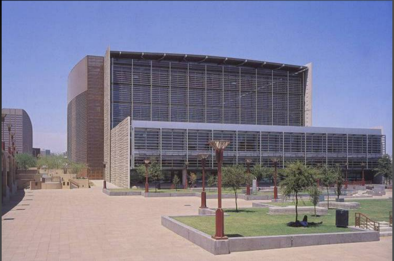
South facade with operable louvers, Phoenix Central Library Will Bruder Architects
