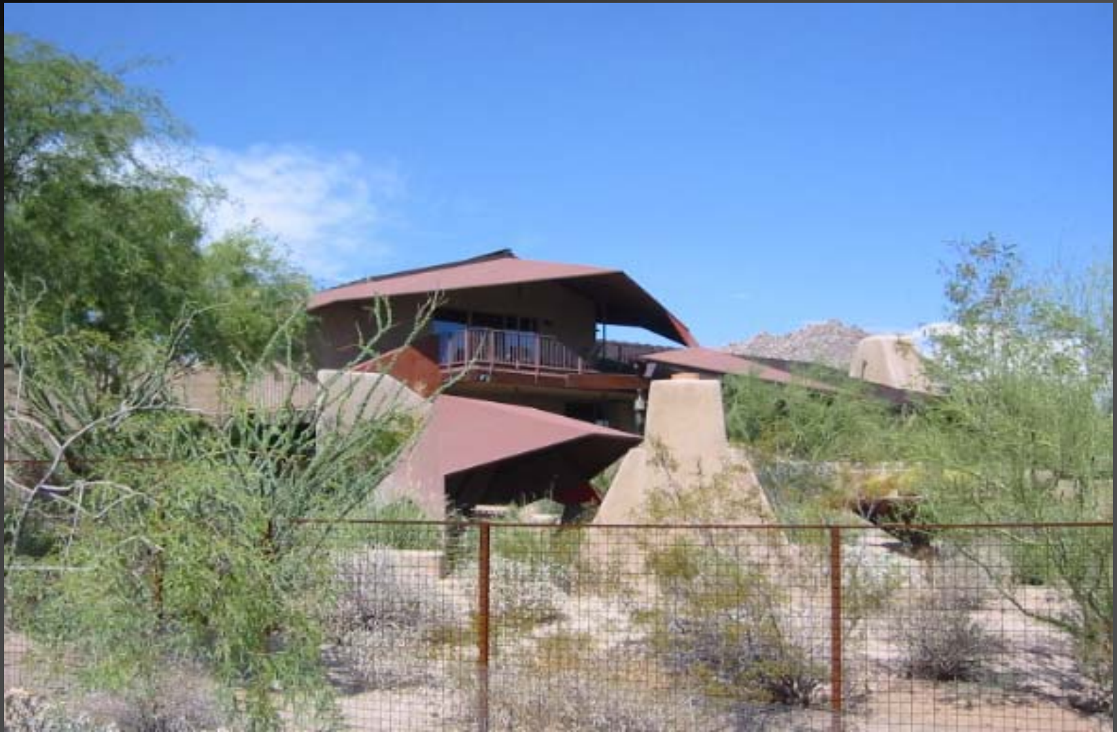
South Elevation in August Swaback Residence
