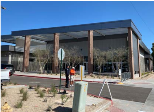
Completed Scottsdale Stadium Renovations
