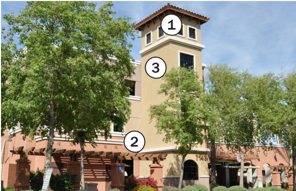
5th Avenue public parking garage.
