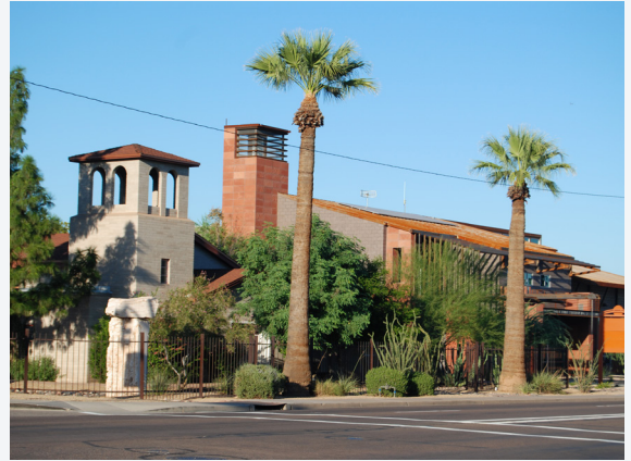
The balance between the new building design of the fire station with the existing church design (foreground) is strengthened by shared features such as concrete block as a key material, tower and roof features with similar geometry, similar roof pitch, street continuity, and metal picket fencing.
