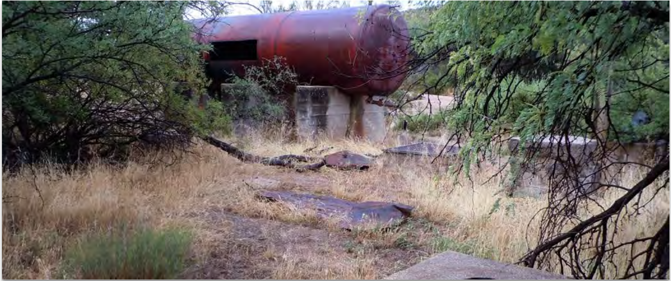
FIGURE 17. HISTORIC WATER COMPLEX AT BROWN'S RANCH.
