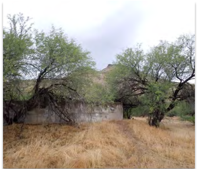
FIGURE 16. HISTORIC WATER TANK (BROWN'S RANCH)
