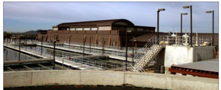
Scottsdale's CAP Water Treatment Plant
